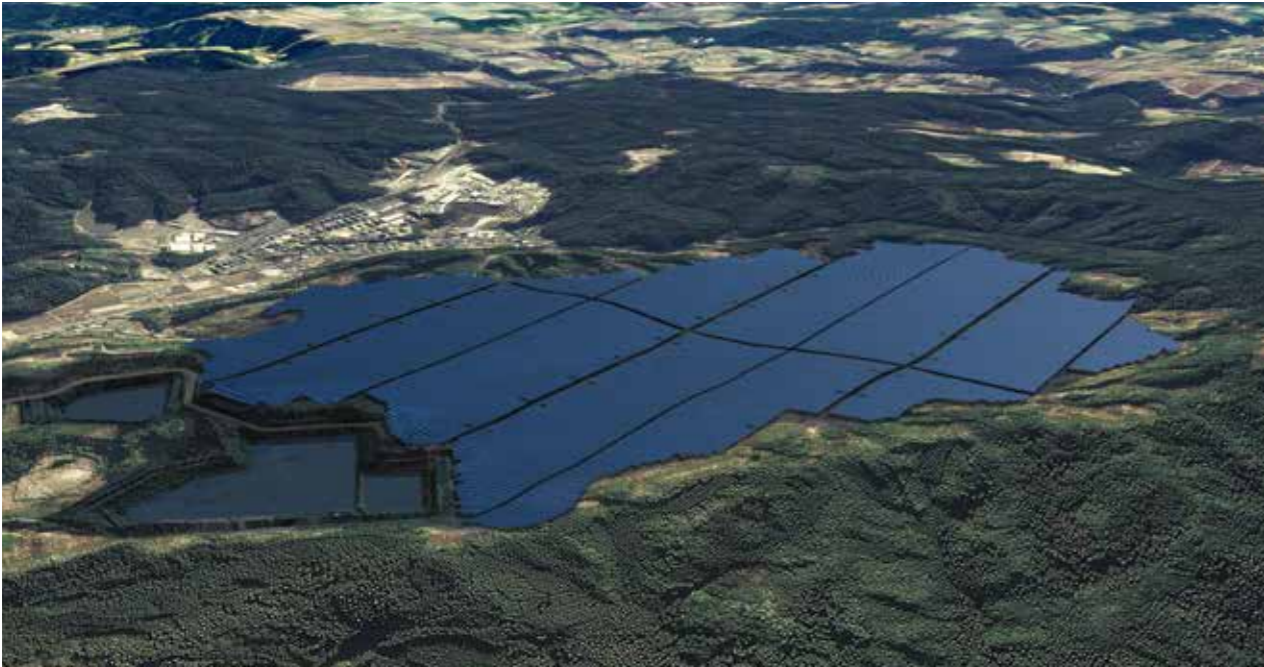
Miyazaki City, Miyazaki Prefecture, Japan 96.2MW / Tallmax / 2018
